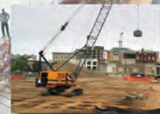
Deep Dynamic Compaction Eliminates Need for Piles
