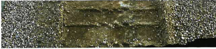
Figure 3: Crawlerway road after the CT has passed over. This shows the effect on the crawlerway, but it was determined before the survey began that the movement of the CT could affect elevation anywhere in the zone of influence.
