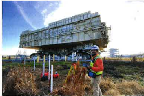
Figure 8: The monitoring process. Top-left: Langan survey crew in position ahead of the CT, prepared to monitor once the CT moves within range. Top-right: CT being monitored from a control point setup within the zone of influence. Lower-left: One member walking with CT calling out station marks, one at total station taking measurements to the prism mounted to the CT, one at the instrument recording data in shared spreadsheet on a field tablet, one using a level placed outside the CT zone of influence to monitor the ground underneath the total station. Lower-right: Station markers were set every 50 feet along the entire length of the crawlerway.
