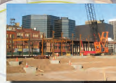
Upgrade in Bearing Pressure Reduces Footing Size
