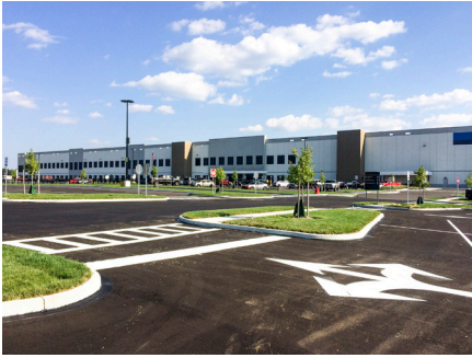
Project Goliath, Fulfillment Center, North Randall, OH
