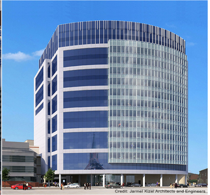
Credit: Jarmel Kizel Architects and Engineers
